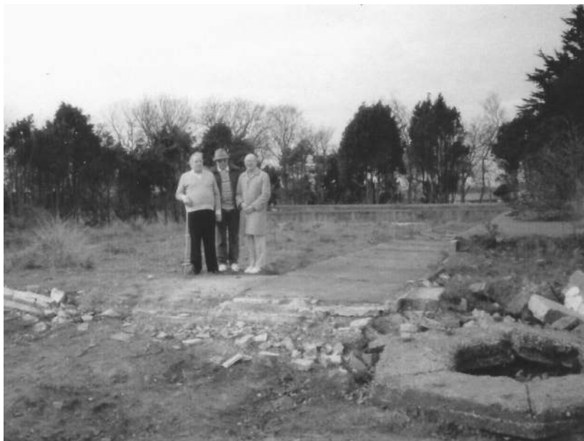
A group of ex-pupils survey the site after the demolition (1990)
